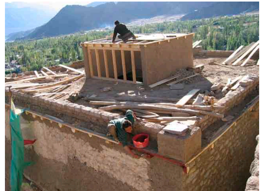
Guru Lhakhang, ground plan and east elevation (THF 2004-2005). Below: the entire roof has been reconstructed, on the picture shown here Ladakhi artisans work on the new rooflight and the parapet.
