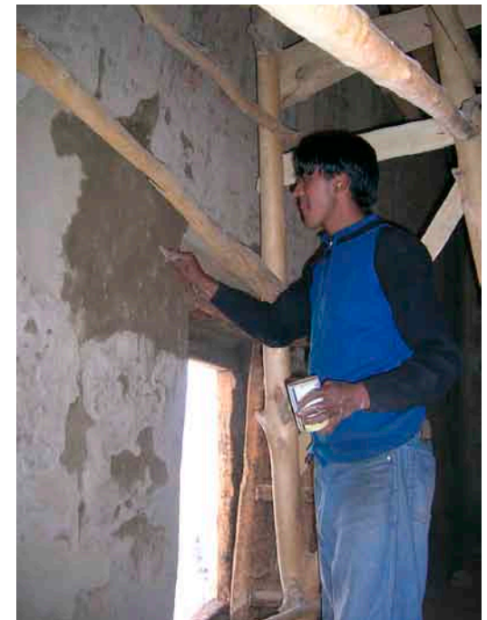
Bottom: Skarma cleaning leakage residue from the east wall.
