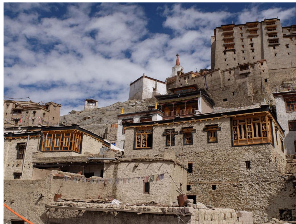
The Kushu (left) and Dzomskit houses after repair, with the Leh palace in the background
