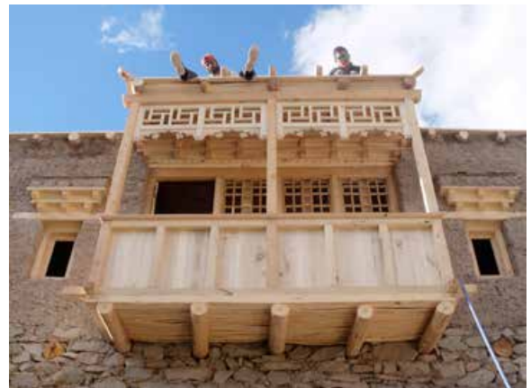
Fitting the Rapsel balcony to the building.
