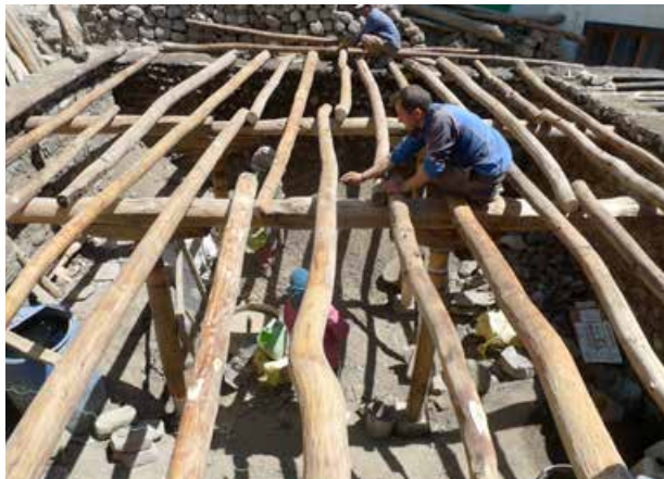
Laying rafters and preparing for roofing work.
