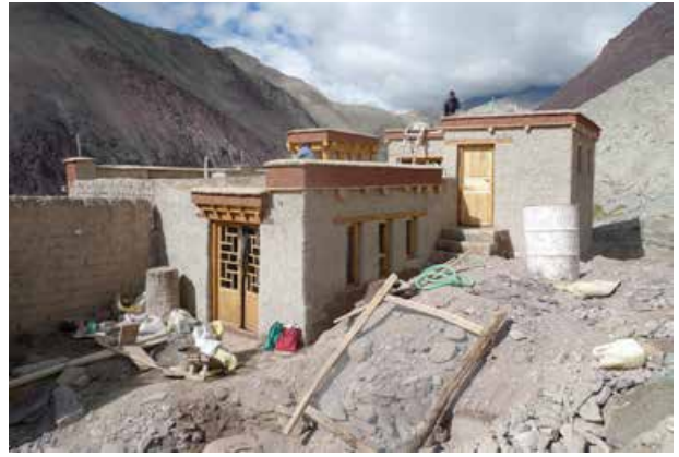
Finalizing work in progress at the rooftop. The building exterior was painted with Markalak whitewash and oxidized iron red.
