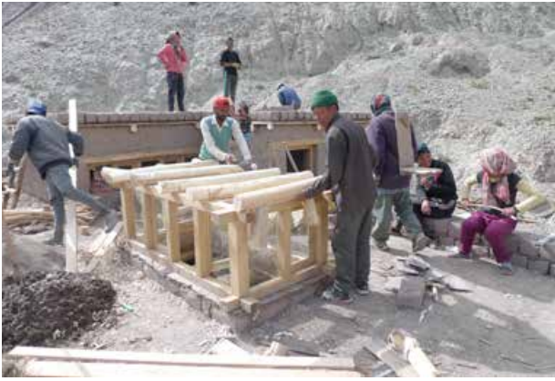
Making a sky-light for the dining room. Very busy rooftop with the working team and villagers.
