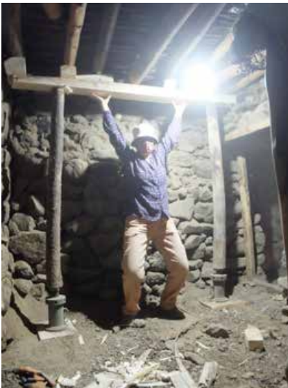
Pimpim lifts up the ceiling structure with help of the jacks.
