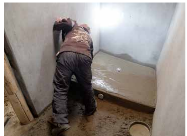
Making platform for shower capsule installation.
