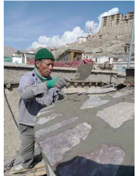
View of the work at Stagophilok Kagan Chorten (stupa) top level. The most vulnerable areas prone to water infiltration were sealed with slate stones. The thirteen rings were consolidated and painted.
