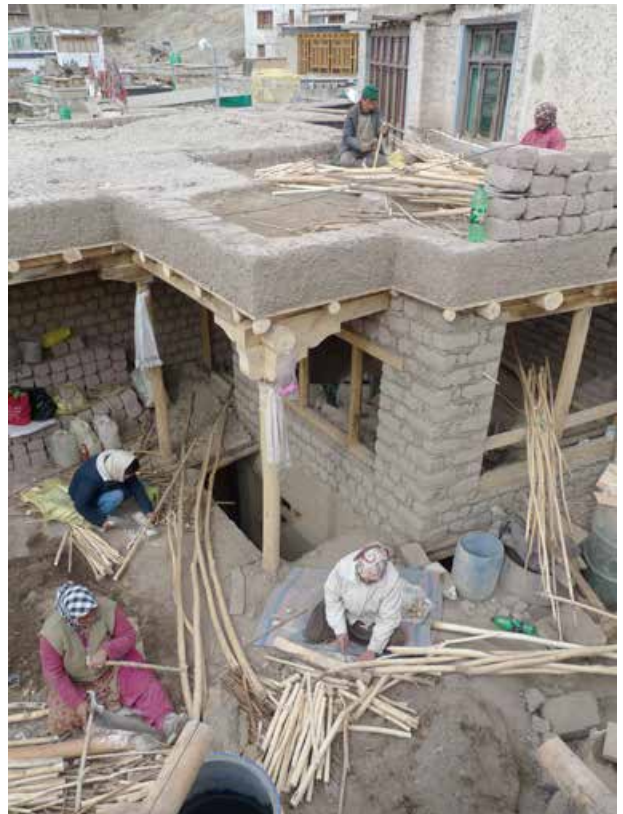
Ladies cutting Taloo willow twigs to prepare for roofing. The staircase opening was covered with a gallery. Main structural works of Bailay house was completed in 2019.
