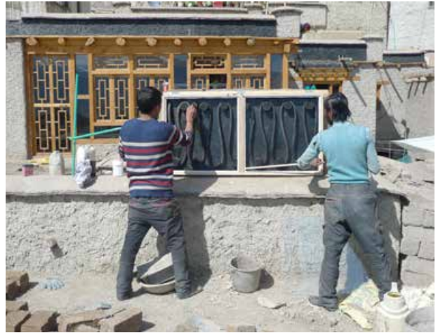
Fixing the glass panel for the insulated water tank storage.
