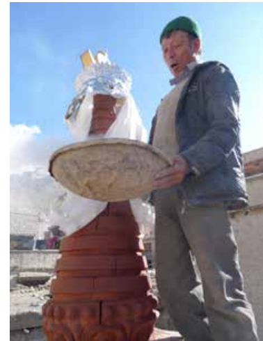
View of the work at Stagophilok Kagan Chorten (stupa) top level. The most vulnerable areas prone to water infiltration were sealed with slate stones. The thirteen rings were consolidated and painted.
