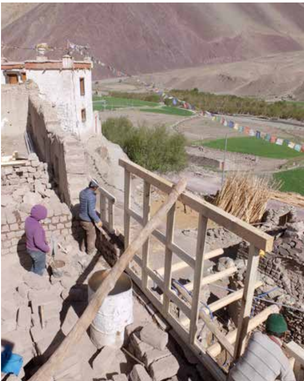
Setting the window frames at the first floor.
