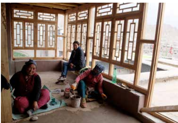
Polishing the mud floor with river stone.
