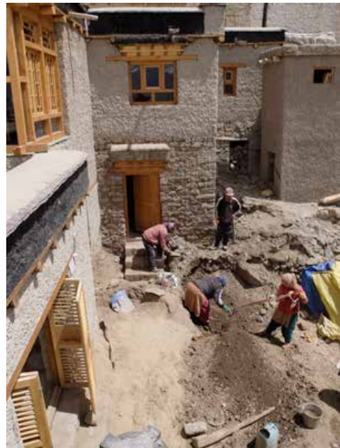
Leveling the ground in preparation for slate stone paving.
