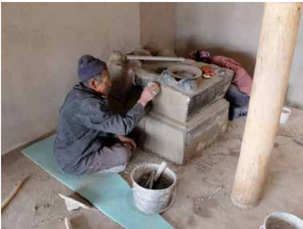
Repairing the original clay stove 'Thab' with special clay.
