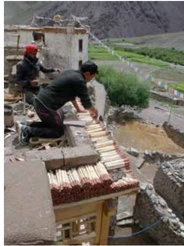
Making a sky-light for the dining room. Very busy rooftop with the working team and villagers.
