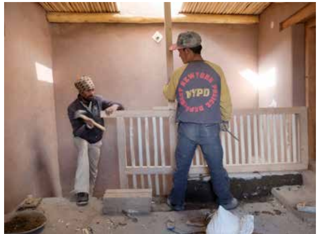
Fixing the railing at the access hall.
