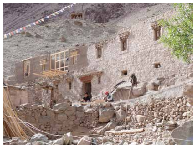
Window frames were fixed in the building, carpenters are preparing more parts for the Rabsel balcony.
