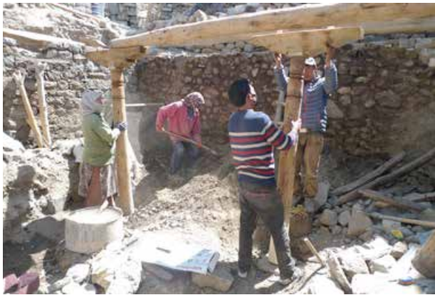
Re-assembling the wooden structure frame in the traditional kitchen.
