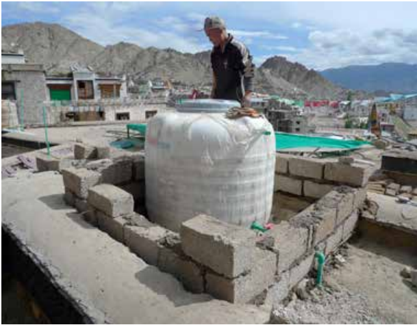
Construction of the water tank insulation wall with saw dust bricks.
