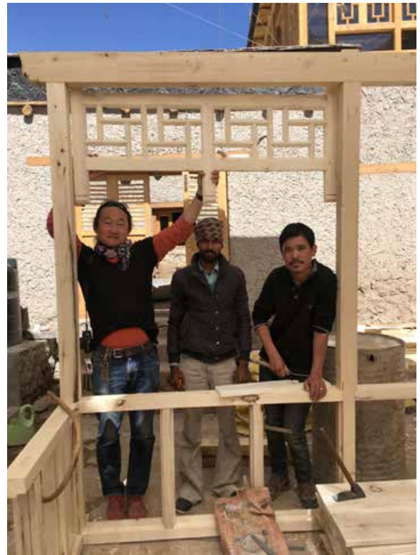
Pre-assembling the Rapsel balcony frame in Leh, the carpenter Rupesh and Dadul made it according to Yutaka's design.
