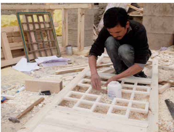
Carpenter is making the latticed door panel, which was designed to integrate with the original window shutter (Seeing on the backside).
