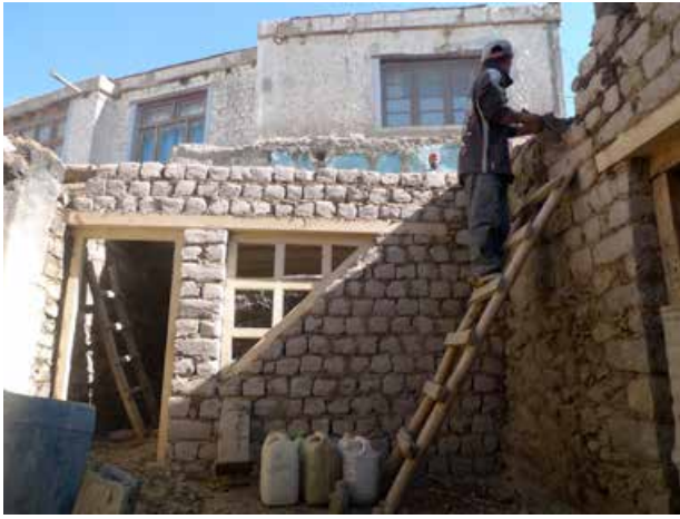
New triangle window was designed to fit with the staircase.
