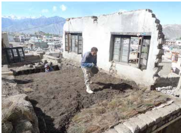
Covering the floor with soil above the Yakzes grass.
