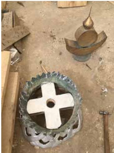
The carpenter repaired the top decoration before putting it back on top of the thirteen rings.
