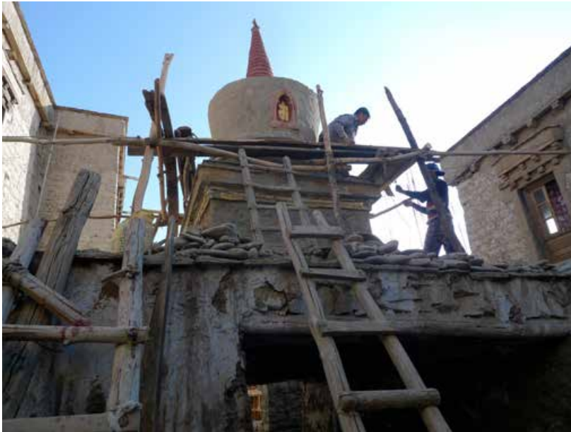
View of the work at Stagophilok Kagan Chorten (stupa) top level. The most vulnerable areas prone to water infiltration were sealed with slate stones. The thirteen rings were consolidated and painted.
