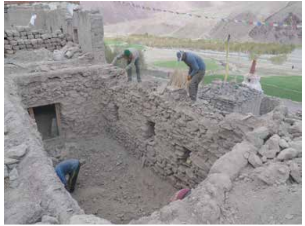
Removed the ceiling structure and preparing to repair the stone wall.
