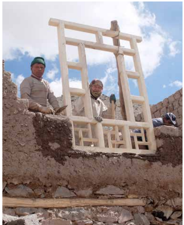
Mason is fixing the newly designed window.
