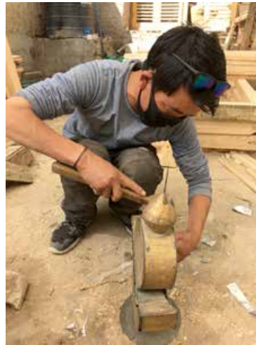
The carpenter repaired the top decoration before putting it back on top of the thirteen rings.
