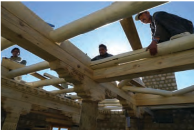
Master carpenter Tsering Dorje and his team laying the roof beam grid. Below: the museum in May 2011.
