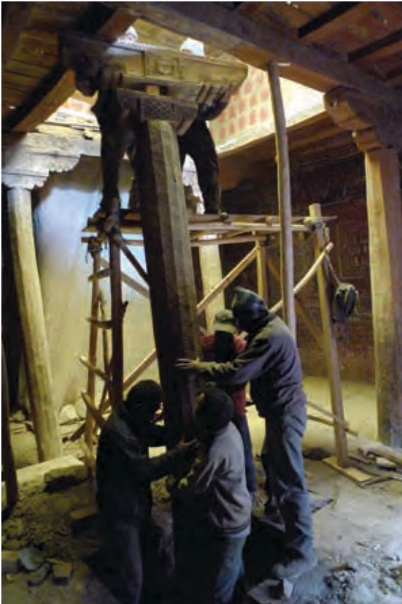
Experienced THF carpenters correct structural settlement in the Chenrezig Dukhang.
