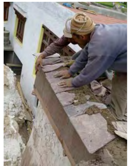
Top: facade of the restored Lama Room with reconstructed stone stairs. Below: restoration of the parapet of the Stupa Hall.
