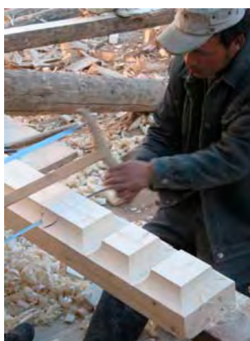
Left: Amdo carpenter preparing replacement dougong brackets. Far left: repair of the outer walls.
