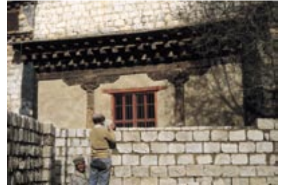
In 1993, the west elevation was permanently blocked by the construction of a public toilet and housing blocks (1993 AA).
