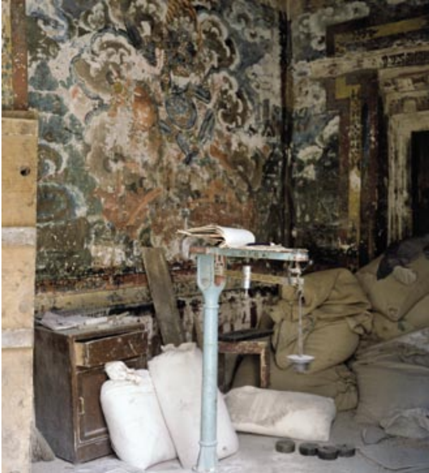
The south portico is used to weigh grain. On both sides are doorways leading to the other ambulatory passage. The 19th century murals are in reasonable condition but in need of some conservation work. Behind the scale is a depiction of Palden Lhamo riding on a horse (1996 AA).
