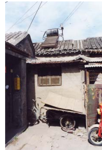
Simple solar shower system setting on the roof
