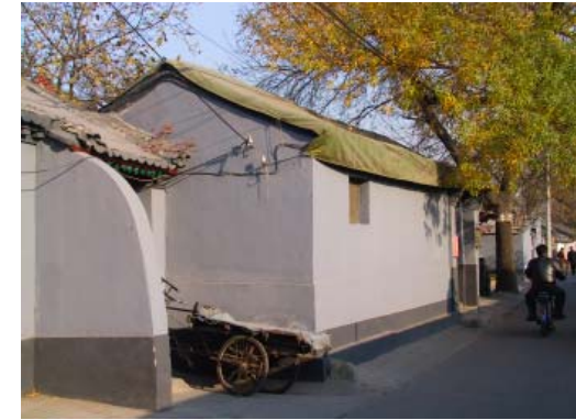
Roof covered by waterproof sheet, lack of technical knowledge for proper maintenance
