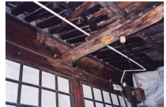
Timber structure damaged by roofleake, in many cases structure problems caused by water and humidity
