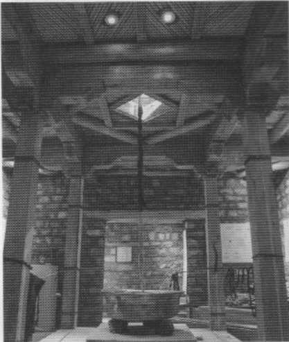
The diamond ceiling allows natural light through all the floors.
