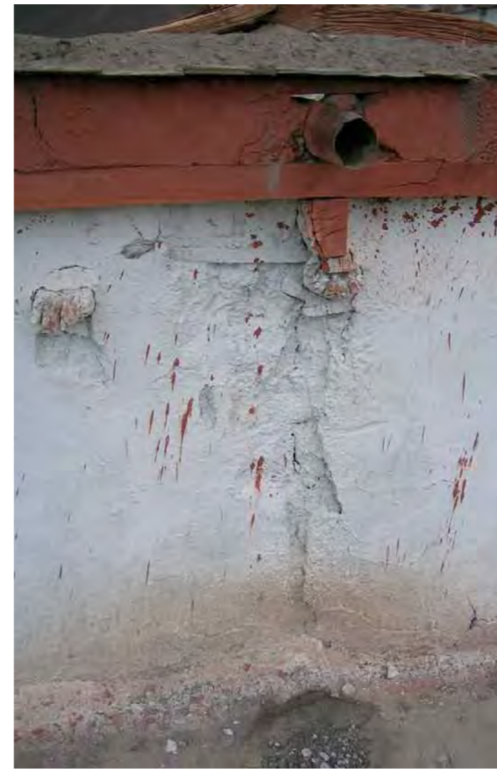
Roof drainage of Dukhang
