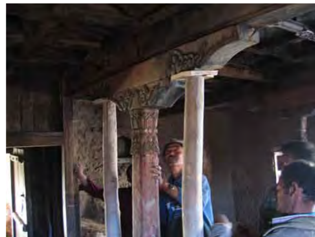
Restoration of historic timber frame, Sofi House
