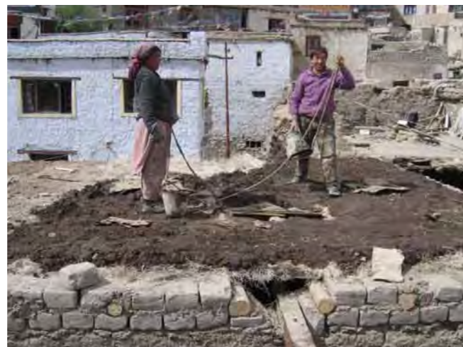
Traditional roof water-proofing, Sofi House
