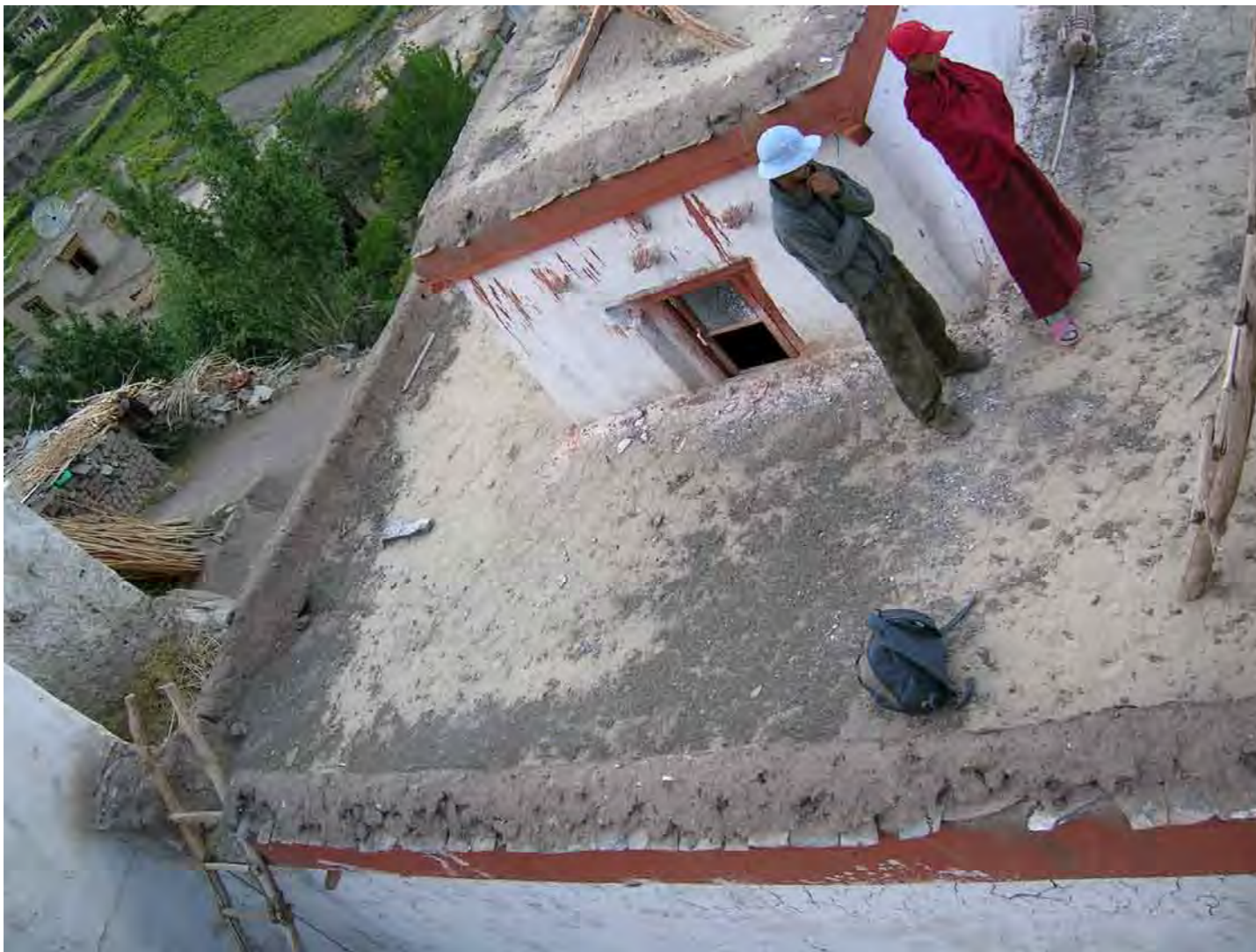
Roof of the Stupa hall
