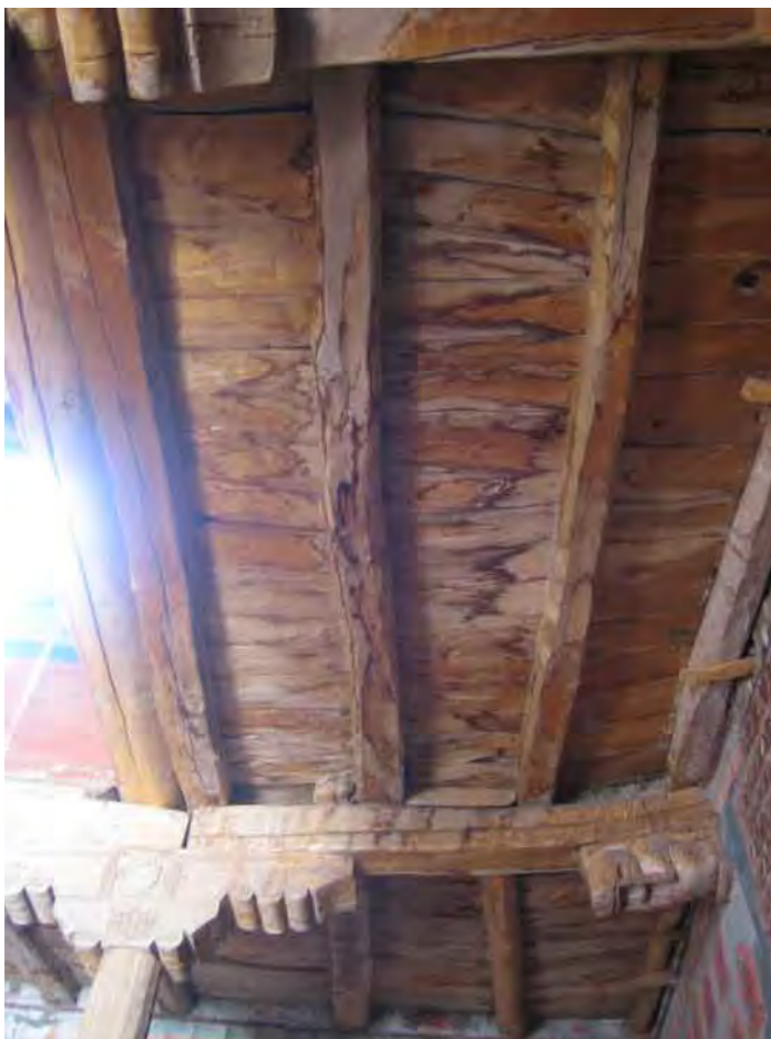
Ceiling, beams, lion brackets and capitals, Dukhang 2nd floor level
