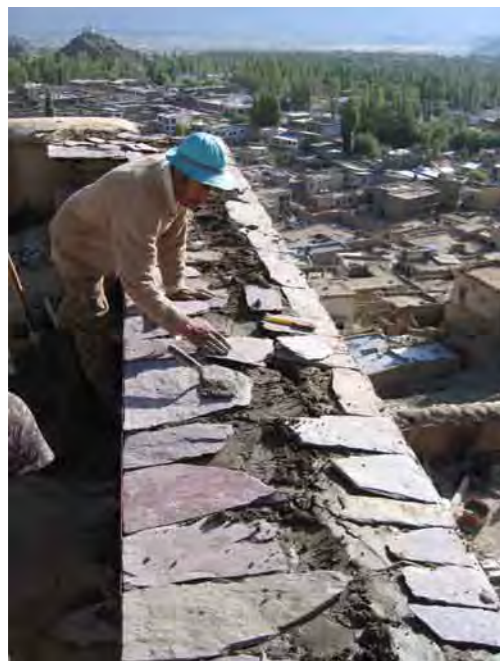
THF builds new parapet, Leh
