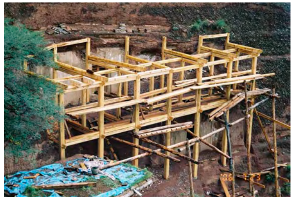
Below: erection of the timber frame and building of Amdo-style tiled roof.
