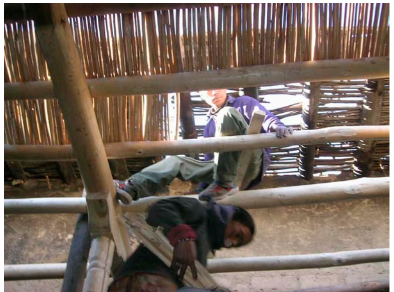
Top: Sankar House at Manikhang, work in progress May 2006; new ceiling structure for the exhibition room. Bottom: Sankar House 1931; same view September 2006.
