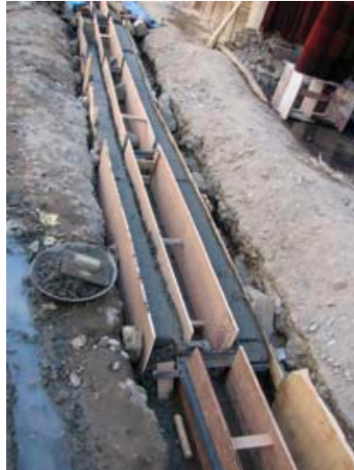
Top: how to build a drain in 3 steps: dig down the concrete road, make a concrete channel and cover it (removable).
