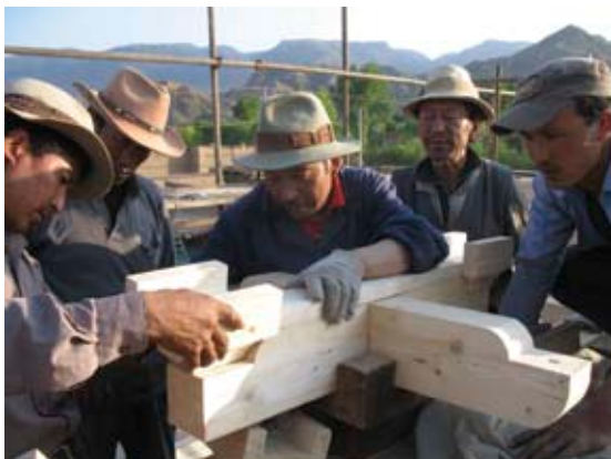
Top: Serkhang monastery. Below: carpenters from Lhasa and Amdo replacing dougong bracket.
