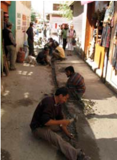
Top: how to build a drain in 3 steps: dig down the concrete road, make a concrete channel and cover it (removable).
