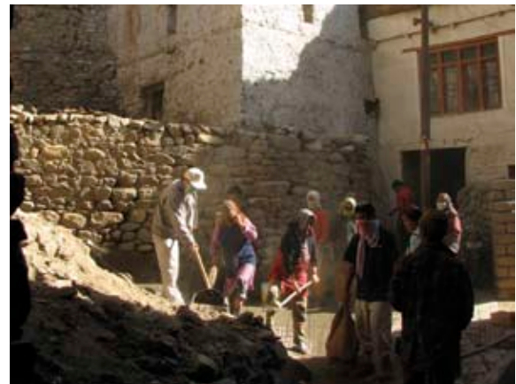
Top: how to build a drain in 3 steps: dig down the concrete road, make a concrete channel and cover it (removable).
