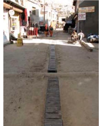
Top: how to build a drain in 3 steps: dig down the concrete road, make a concrete channel and cover it (removable).
