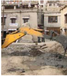
Left: the open foul-smelling cesspool at Manikhang. Top: we hired an excavator to remove tons of semi-liquid waste.
